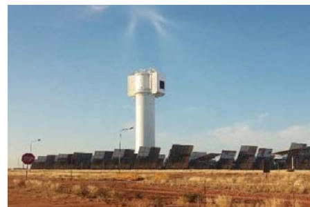
Figure 37 A central tower surrounded by heliostats.
