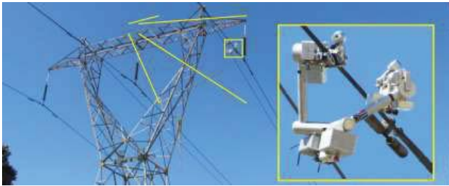
Figure 30 Power line inspection robot navigating around a damper on a 132 kV line.
