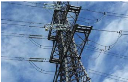
Figure 31 Power line inspection robot climbing from a jumper to the main line on a (220 kV) strain tower.
